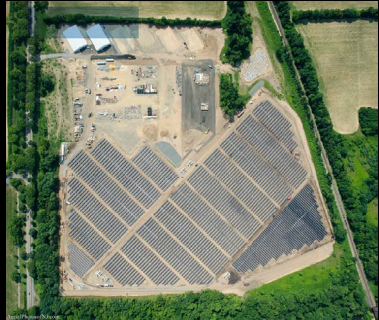
Solar Panel Field (4.5 MW Capable)
